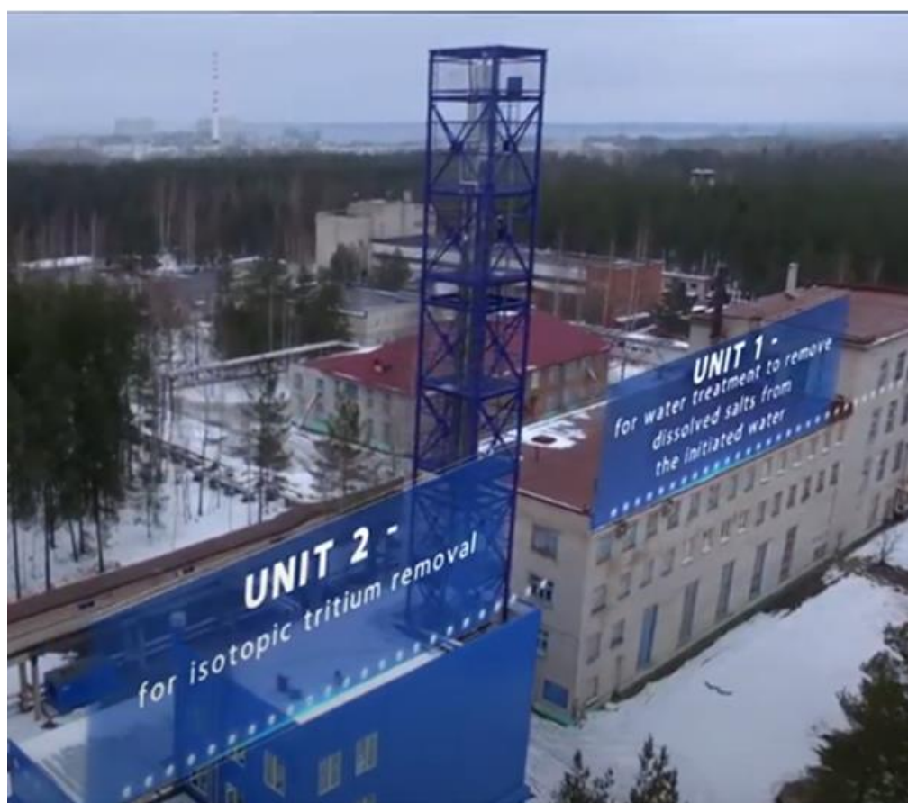
Fig. 10 - Demonstration plant with a rectification column for detritisation of liquid radioactive waste at the Fukushima NPP (Radium Institute, Sosnovy Bor)
